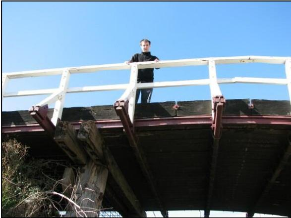
Greg on the bridge. The wooden pylons, bent rail track decking and cross-pieces can be seen. Photos Kevin Phillips.
