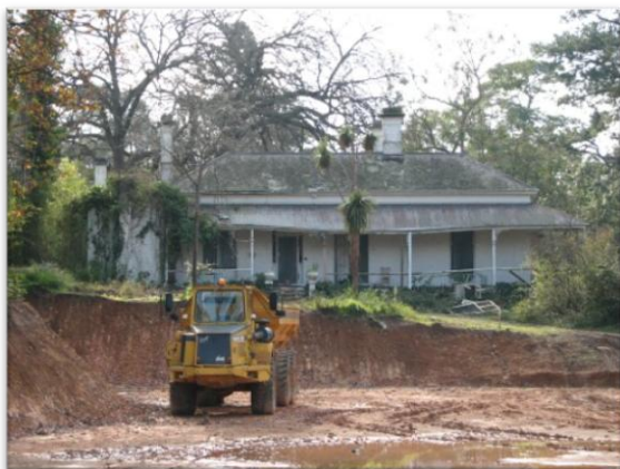
Decaying beauty: derelict house below the Rail Trail, Maroondah Highway, Lilydale.
