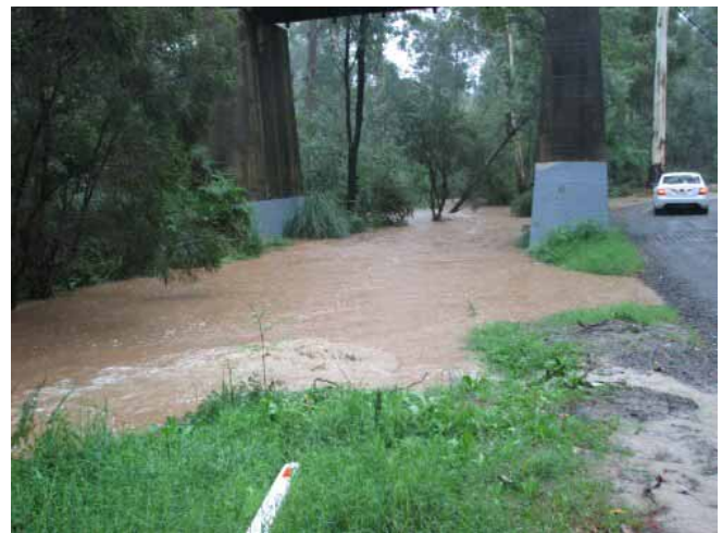
Water under the bridge: the swollen Stringybark Creek laps the pylons of the Rail Trail bridge at Forest Road. Photo Kevin Phillips.
