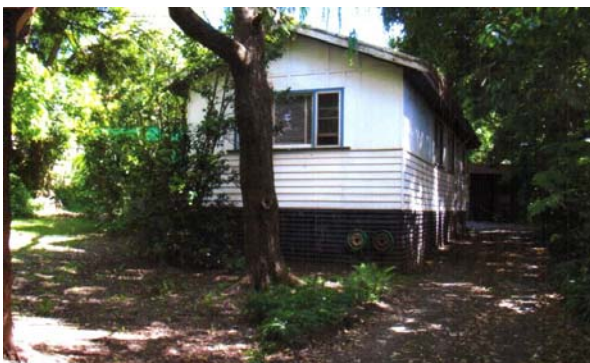
Above, the house Alan built at 9 Silvan Road.
