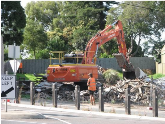
Demolition machinery at work on the old shop, 14/2/2000.
