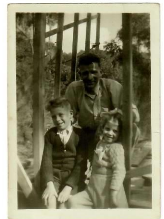
My father, Graeme and I at the Mt Evelyn block in a half completed house.
